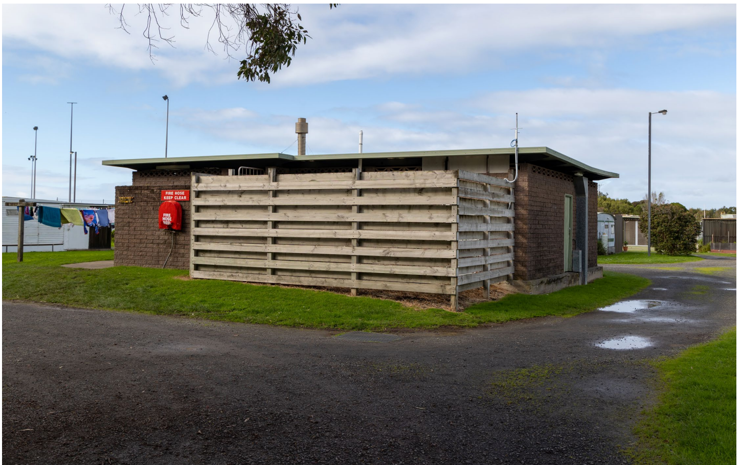
Existing northern amenities building
