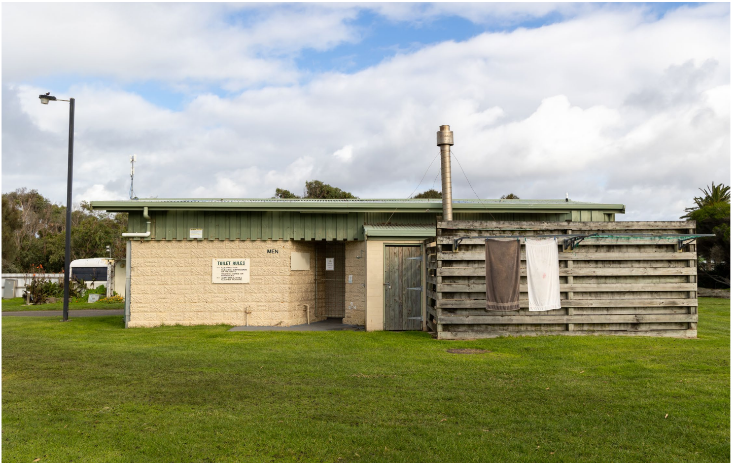
Existing central amenities building
