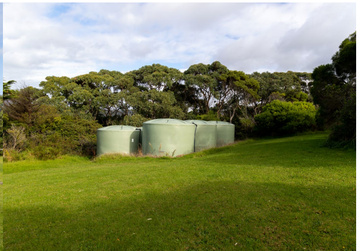
Water storage tanks
