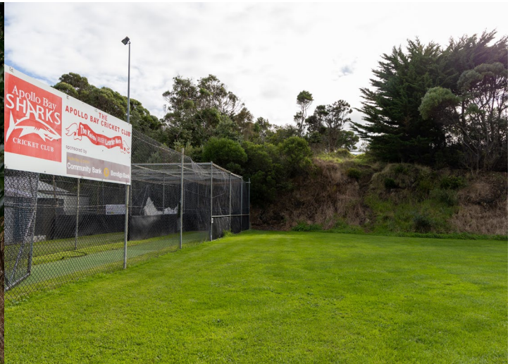
Embankment above cricket nets
