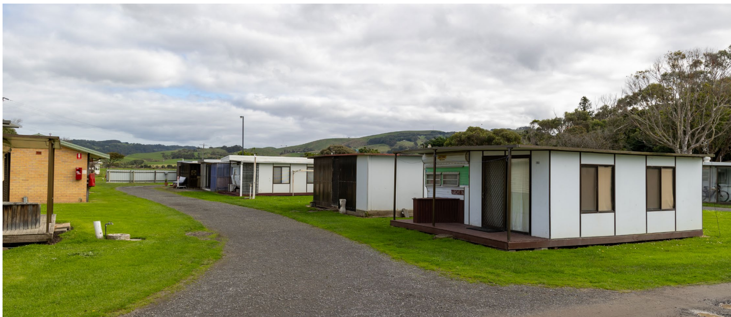
Existing structures built by annual permit holders
