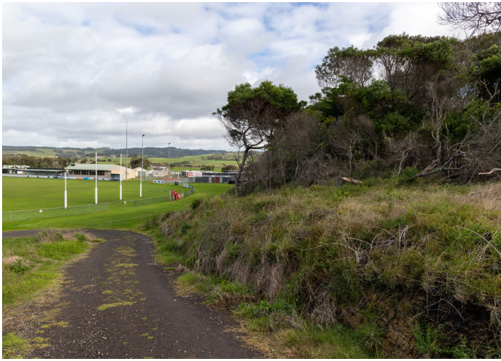
Cleared embankment above oval
