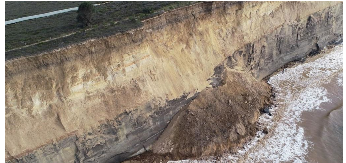
Figure 1 - Cliff failure at Demons Bluff, Anglesea (2019).
